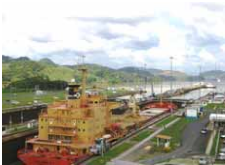
Ship at Miraflores Locks enters the Panama Canal
