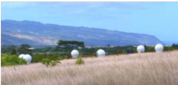
MEOLUT (MEOSAR Local User Terminal) in Hawaii. Installed for the U.S. government in September 2011, it is the first six-antenna ground station of its type in the world. Its 3.7 m antennas track MEOSAR satellites orbiting 22,000 km above the Earth that listen for distress signals.
