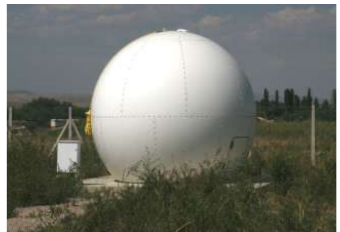
One of two MEOLUT antennas installed in Ankara, Turkey in August 2010. The Turkish MEOLUT is part of a five-MEOLUT network distributed across five countries on four continents — a network currently featuring a total of fifteen MEOSAR antennas to receive and share distress alerts.
